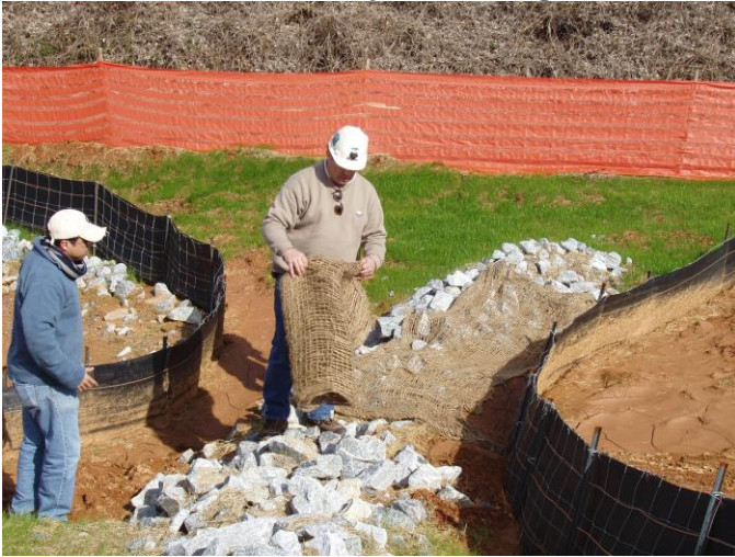
Cover rock check with jute matting
