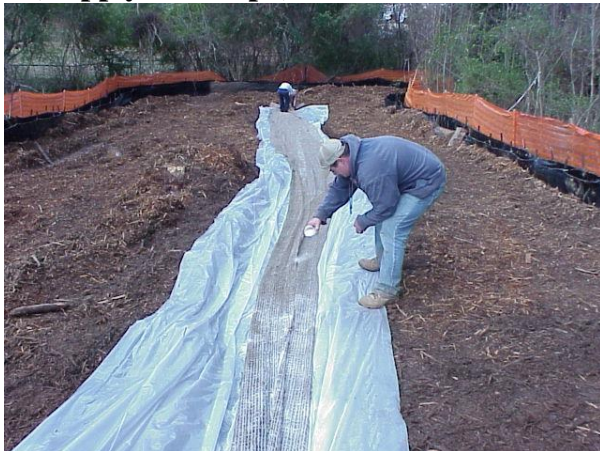
5) Apply Silt Stop (downstream end)
