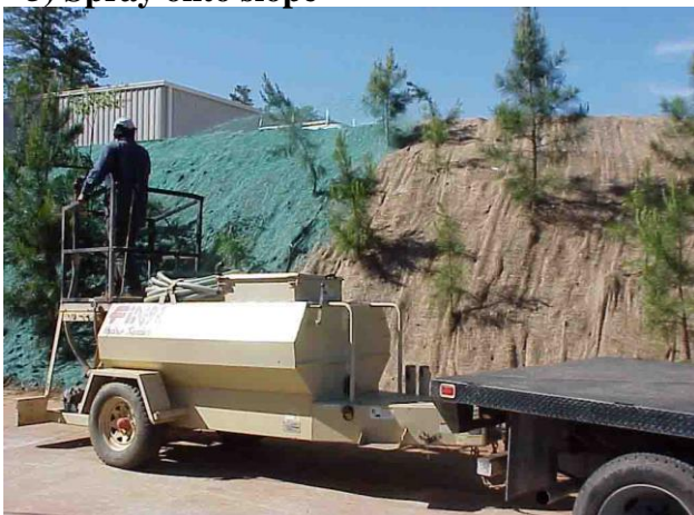
5) Spray onto slope
