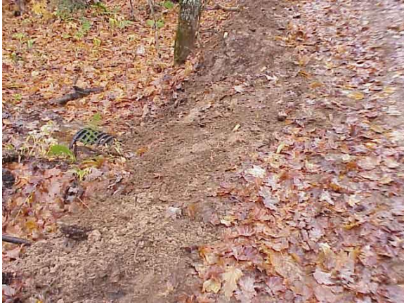
1) Fill rills and gullies
