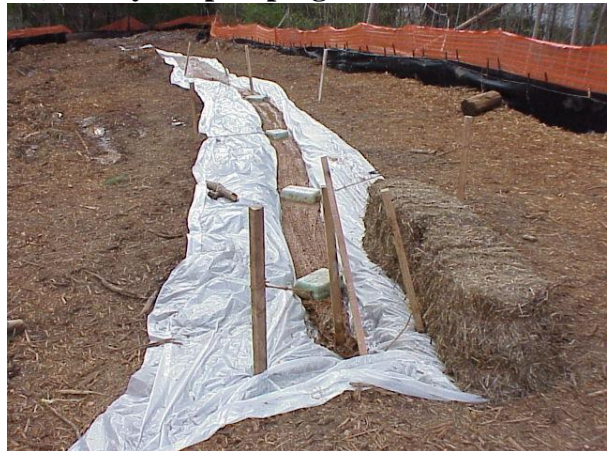
6) Ready for pumping
