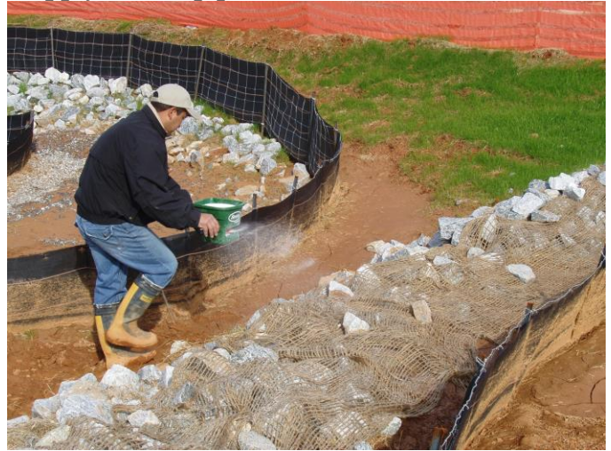
Apply Silt Stop powder over rock check
