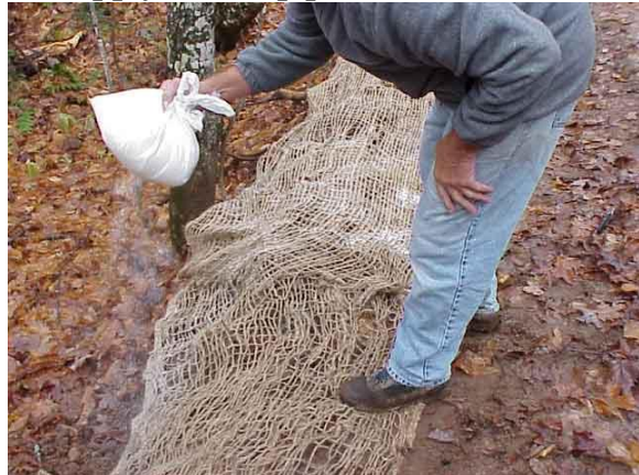
4) Apply Silt Stop powder
