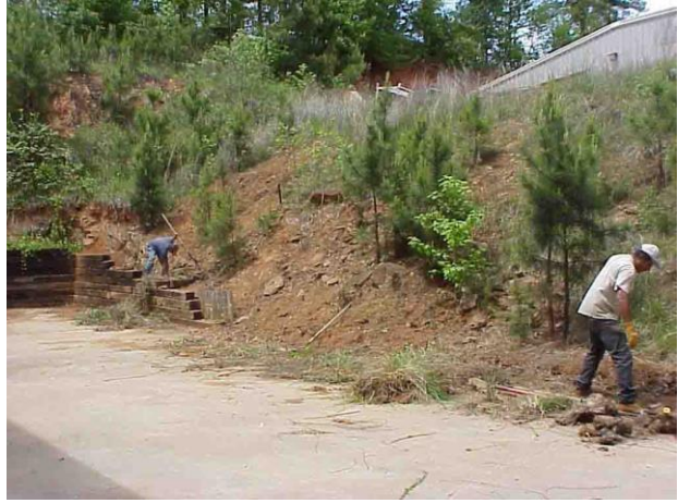
2) Fill rills and gullies
